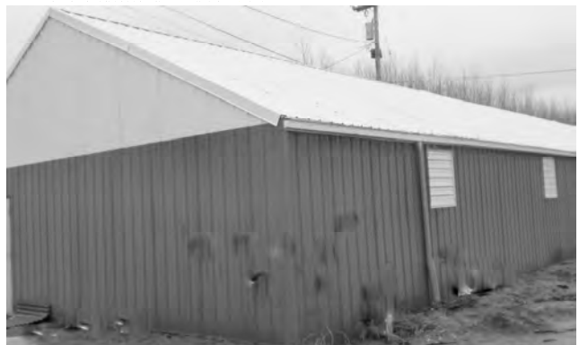
The newly remodeled dog training center nears completion.
